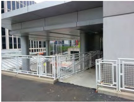
NoMa Access Point - stairwell and elevator
