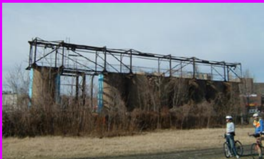
Abandoned silos at Rhode Island Avenue.
