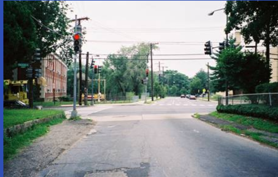
Blair Road/Riggs Road Intersection (A5)
