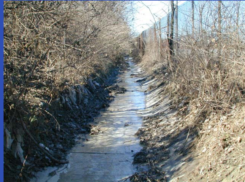
Looking North Along Culvert (A1-A5)
