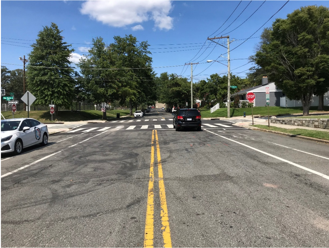
Figure 20: 3 rd Street, NW Northbound Mid-approach
