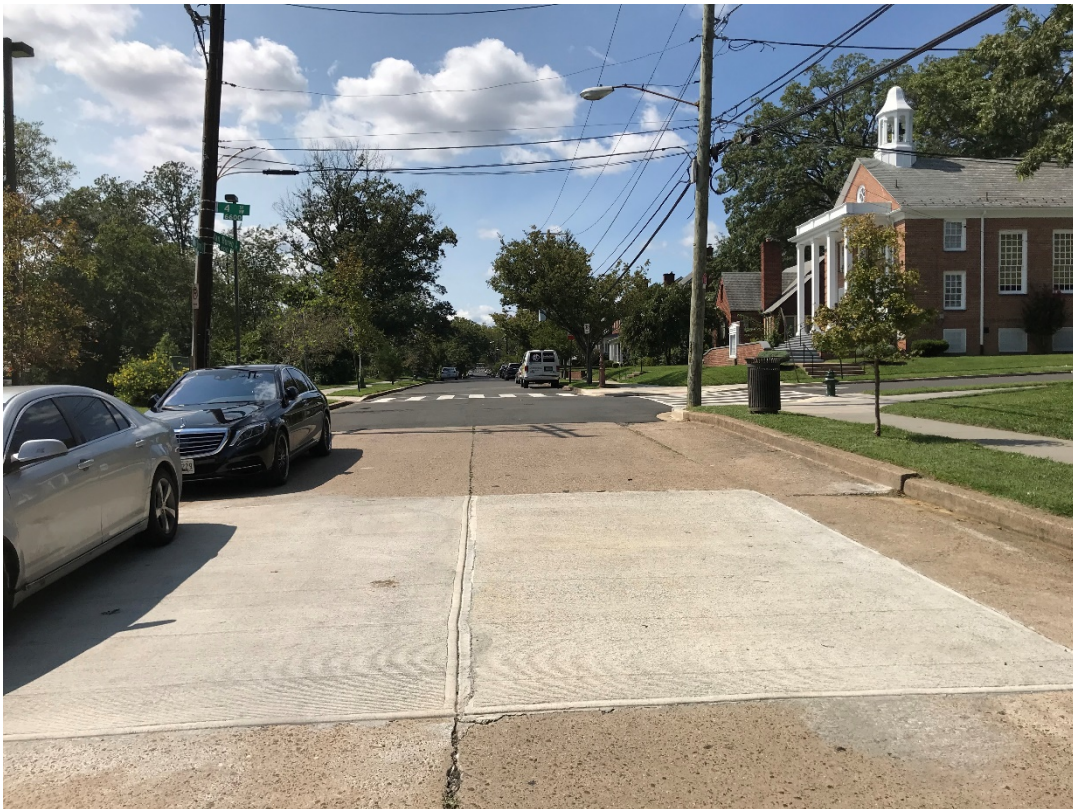
Figure 18: Van Buren Street, NW East Leg Mid-approach
