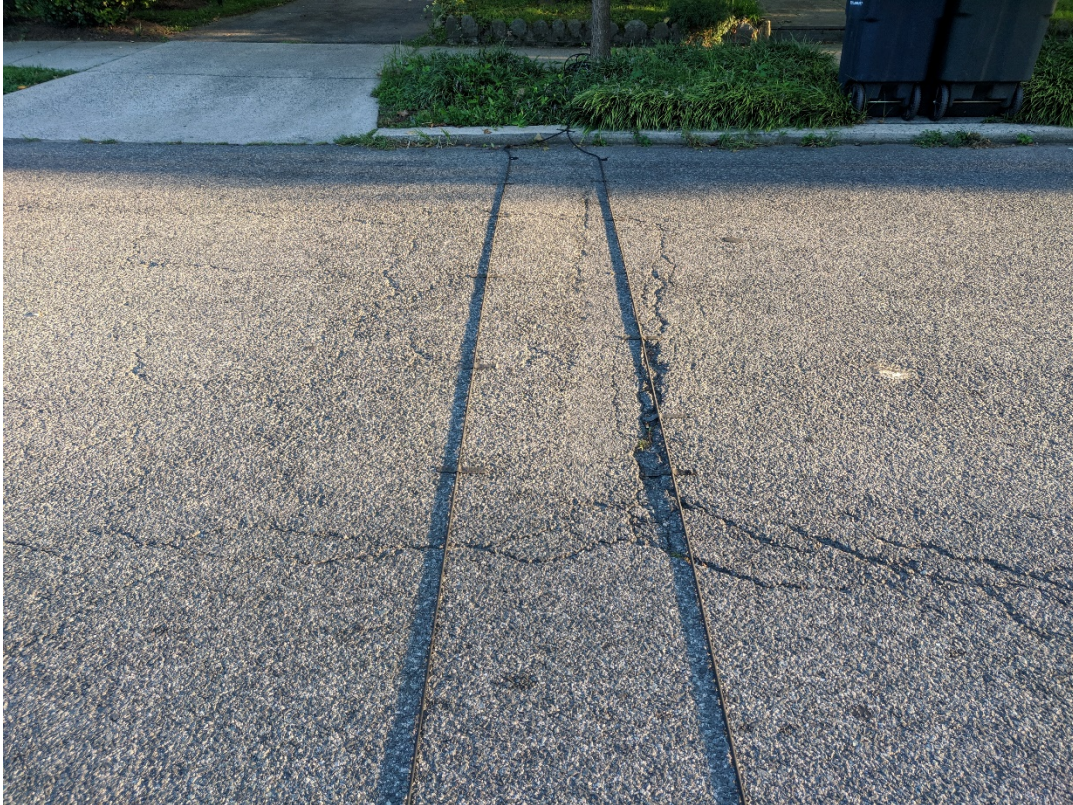
FIGURE 2: Tubes on 300 block of Aspen Street, NW
