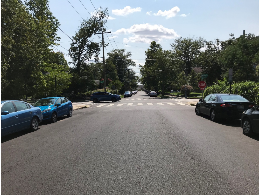
Figure 11: 4 th Street, NW Southbound Mid-approach
