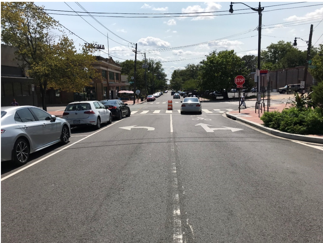
Figure 4: 4 th Street, NW Southbound Mid-approach
