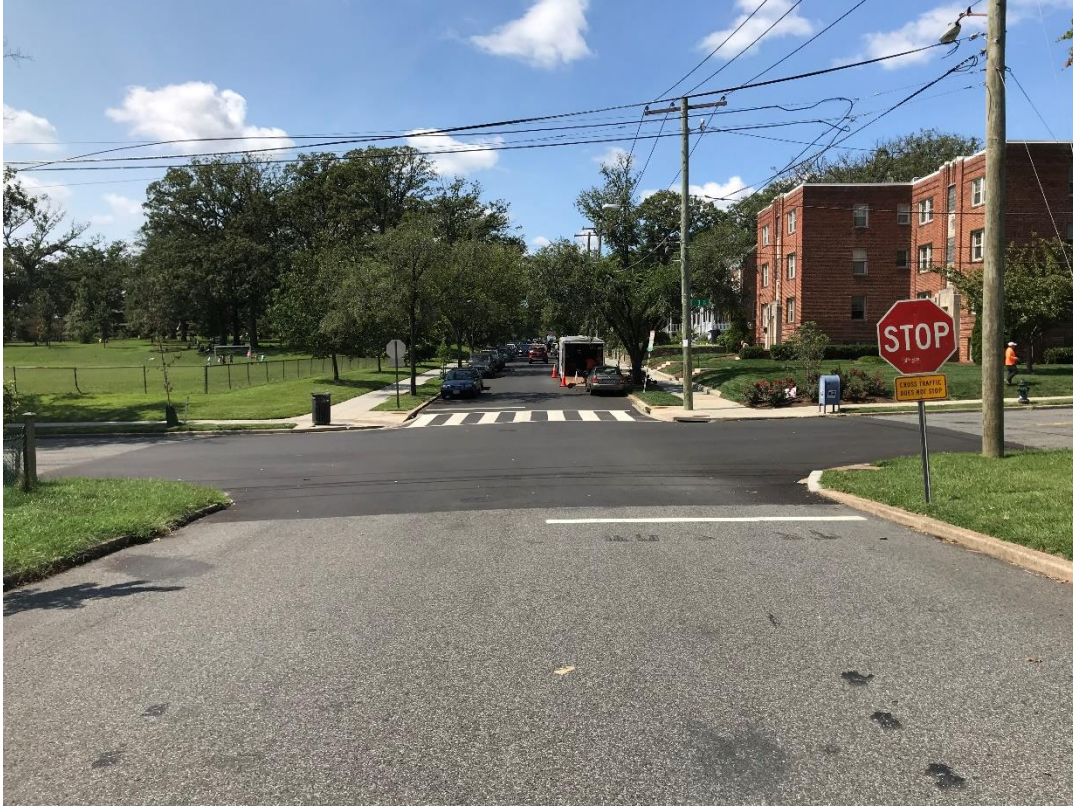
Figure 5: Whittier Street, NW Westbound Mid-approach
