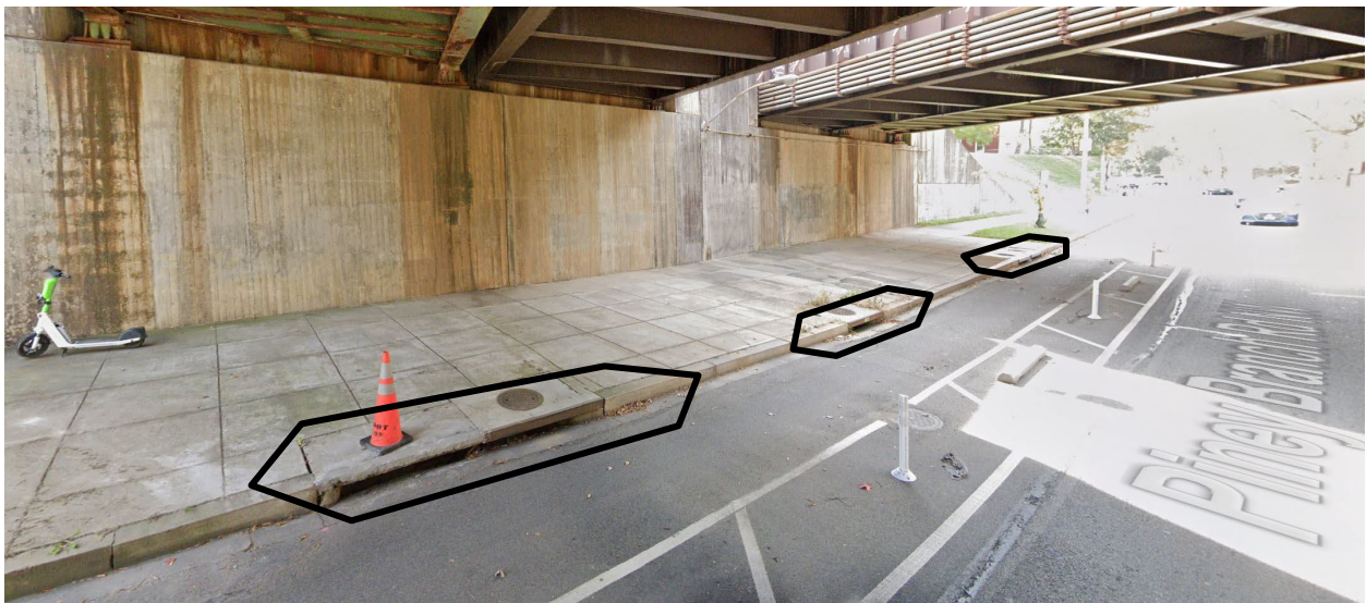
Figure 23. Existing Stormwater Drainage Components – Piney Branch Road
