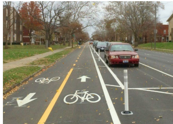
Figure 39. Two-Way Protected Bicycle Lanes
