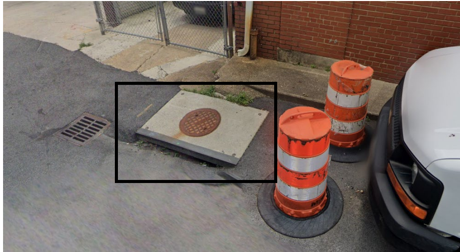
Figure 28. Catch Basin and Field Grade Inlet - Spring Place
