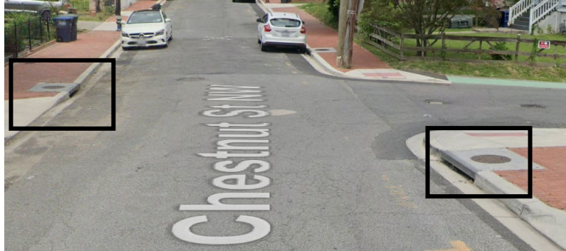
Figure 26. Existing Stormwater Drainage Components – Chestnut Street
