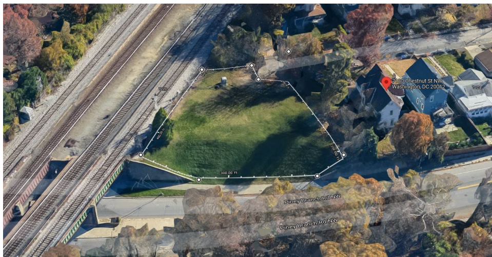
Figure 25. WMATA-owned Parcels – Overhead View
