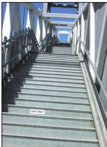
Staircase with Concrete Bicycle Rolling Tray on the Side
