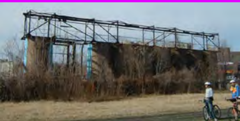
Storage silos near Rhode Island Avenue.
