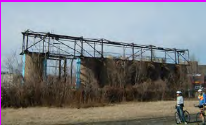
Abandoned silos at Rhode Island Avenue.
