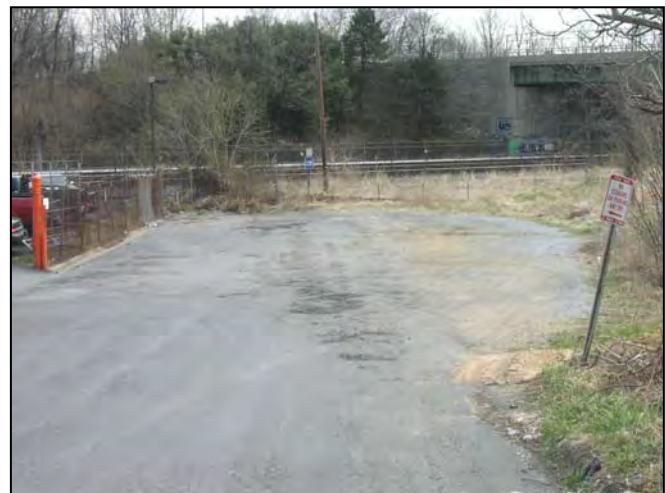
Looking south on Oglethorpe Street toward the CSX underpass
