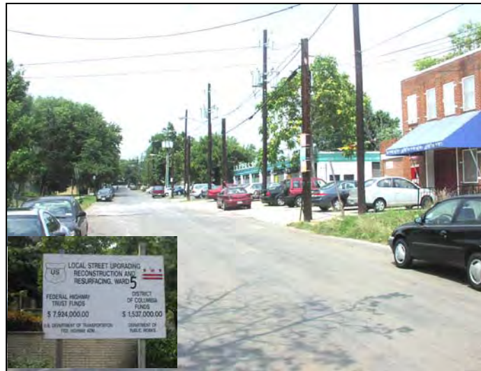
Reconstruction of 8th Street will include completion of a continuous sidewalk on the west side and a shared use street for bicyclists.
