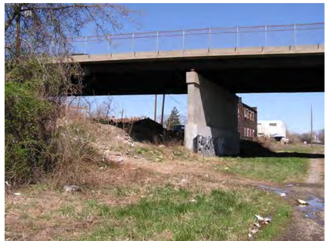
Looking north toward 8th Street at the Franklin Street overpass
