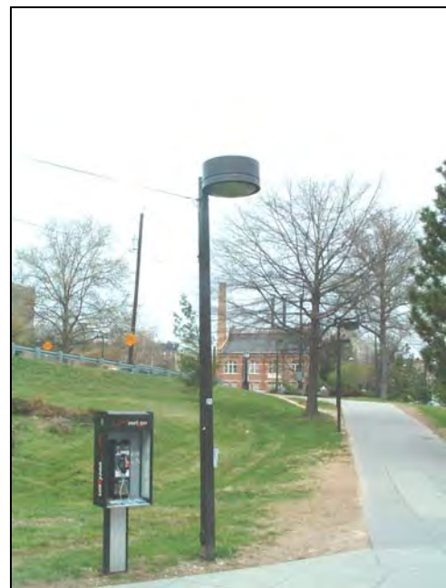
Existing Lighting at the Brookland /CUA Metrorail Station
