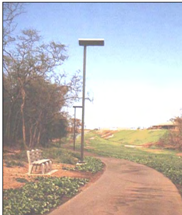
Overhead Photovoltaic Lighting
