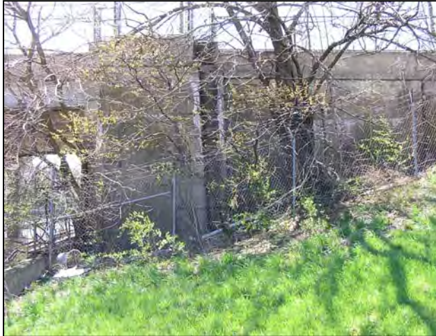
Looking south toward abutment of Monroe Street overpass
