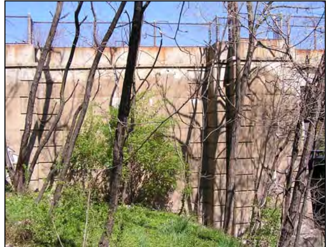
Looking North toward bridge abutment of Monroe Street overpass
