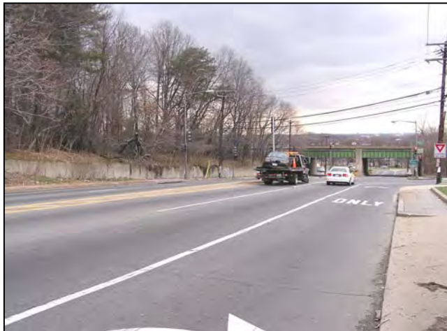
At-grade crossing at Riggs Road/First Place intersection, looking east
