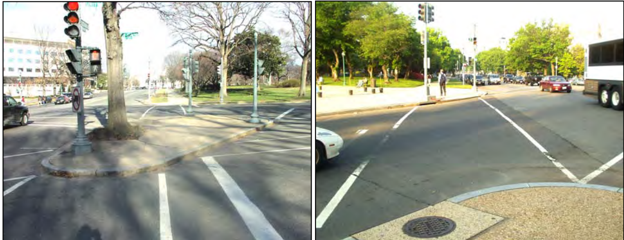
Implementation of the MBT will improve pedestrian and bicycling conditions along Louisiana Avenue, where curb ramps are missing and crossing distances are long. (C and New Jersey on left; D and North Capitol on right.)
