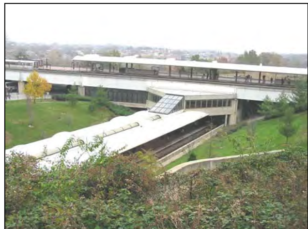
Looking down on Metro Station
