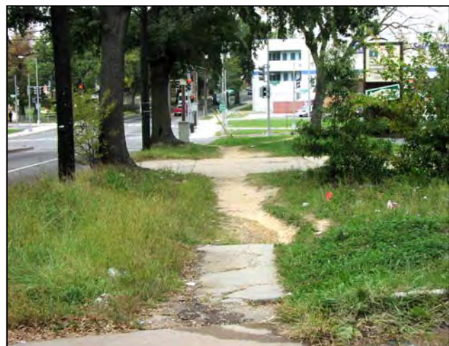
MBT will provide long needed sidewalk improvements on Blair Road.
