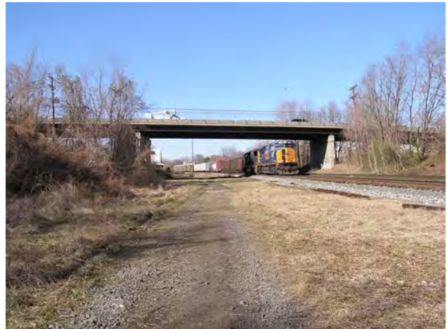
Looking north along CSX right of way
