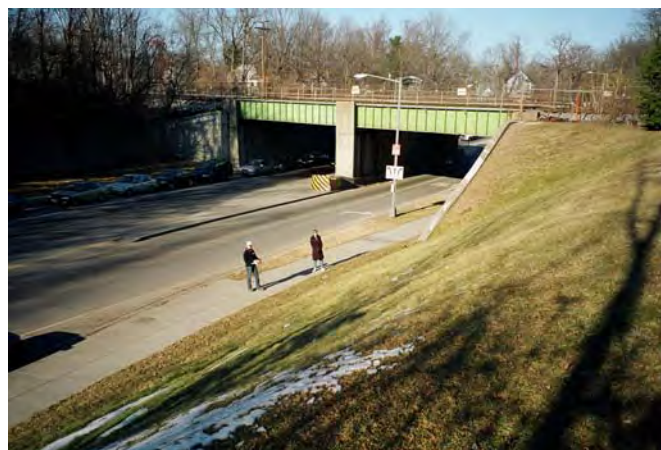
Overpass over Piney Branch Road, looking east
