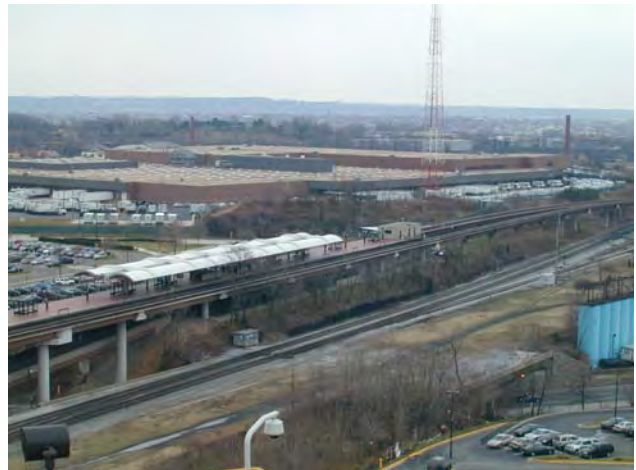
Looking down and south at the Rhode Island Metrorail Station
