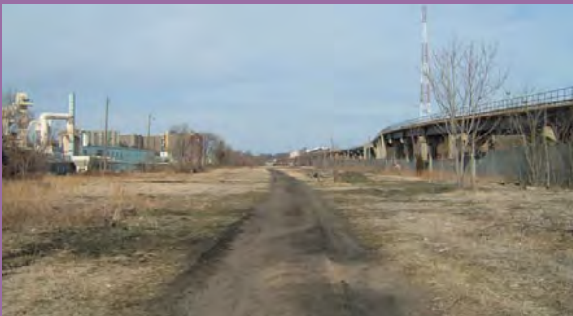
Rail corridor segment, north of New York Avenue.
