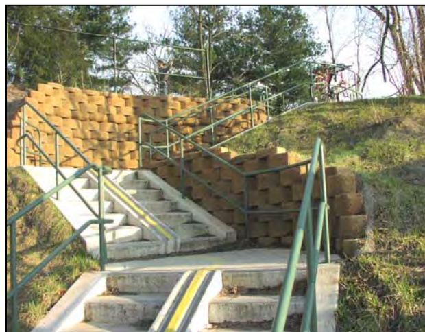
Staircase with Concrete Bicycle Rolling Grooves in the Center
