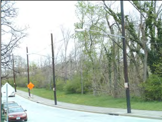
Existing Lighting on John McCormack Road
