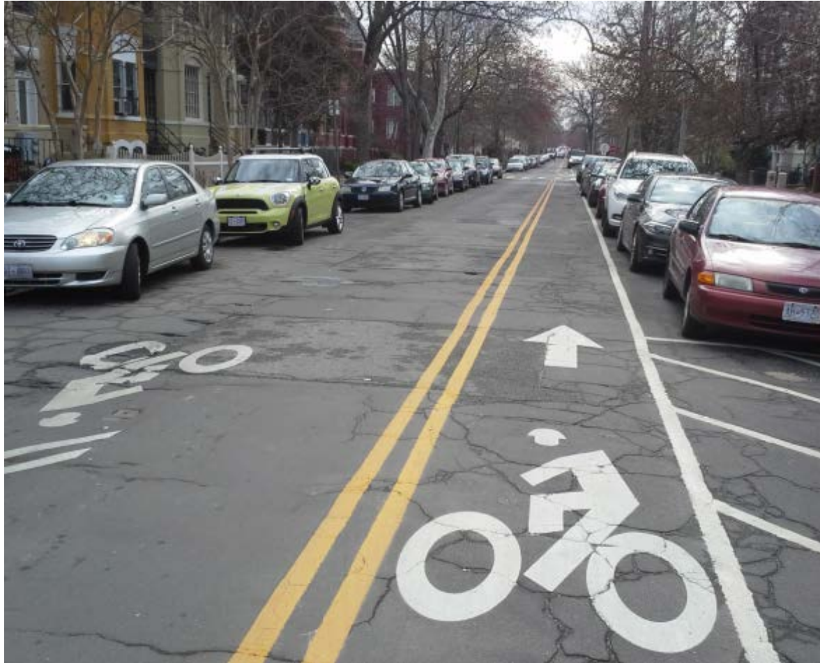
Example of a contra-flow bike lane on G St NE. A contra-flow bike lane is proposed on McDonald Place NE
